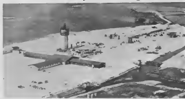
In November 1969 several foundations for HDS units started, including the one for the process stack.
